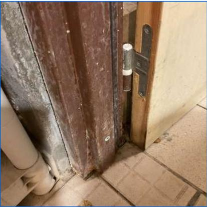
A close-up photograph of a door frame. The metal frame is heavily rusted and shows signs of significant wear and corrosion. The door is partially visible, and the floor is tiled.
