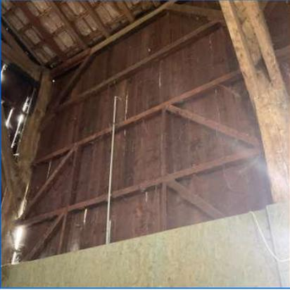
A photograph showing the wooden bracing of a building's long side. The structure is made of dark brown wood and features a complex network of diagonal and horizontal beams. The bracing is used to support the roof and walls. The background shows a wooden ceiling and a wall.
